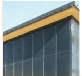
**The Centre d'exploitation des Routes Nationales (CeRN) is a maintenance building of the Swiss motorways. The building is an excellent example of solar thermal collectors integrated into a building façade by adapting an Energie Solaire solar roof system.**
