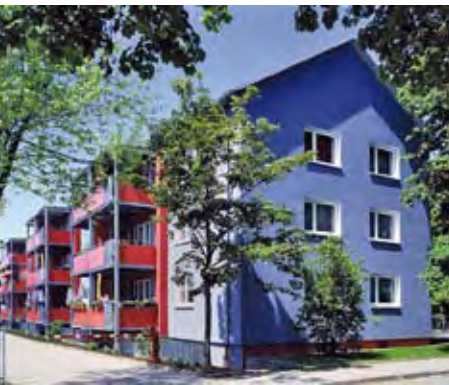
Apartment Building in Freiburg i.B., DE
