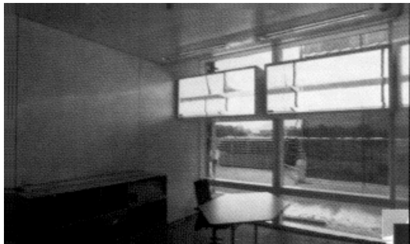
A testroom with an anidolic daylighting system at LESO, Ecole Polytechnique Federale de Lausanne, Switzerland
