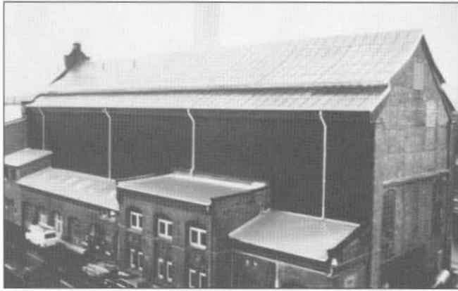
This co-generation plant in Gottingen, Germany, installed the first perforated solarwall in Europe.
