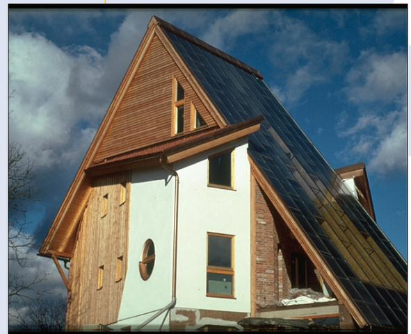
▲ **Figure 1. The first detached house using a solar combi system that covers 100% of the hot water and space heating needs was built in 1997.**
