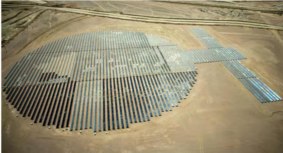
**Figure 12: Flat-plate collector field of 39,300 m<sup>2</sup> at Codelco's "Minera Gabriela Mistral" in the Atacama Desert, Chile (Source: ArconSunmark)**
