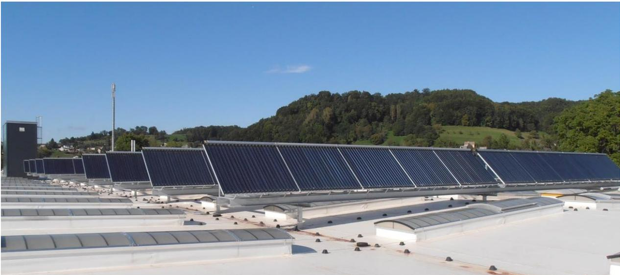
**Figure 13: Field of 80 high performance evacuated tube collectors with CPC reflectors on the roof of Zehnder in Gränichen, Switzerland, with a gross area of 394 m<sup>2</sup> (Source: Ritter XL Solar)**
