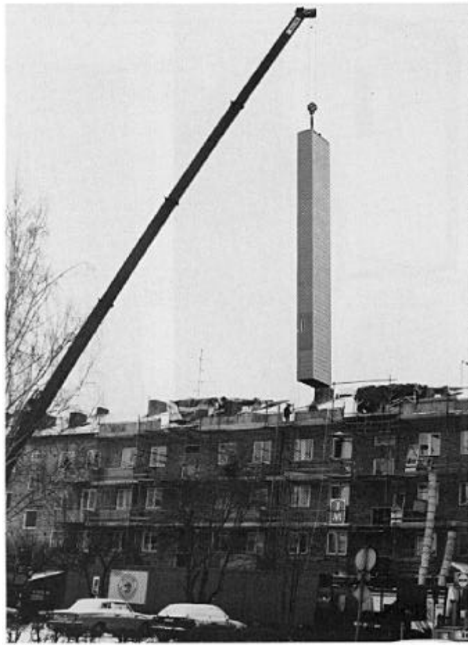
Fig. 4. Rapid lift installation - Completely prefabricated lift shaft [2]
