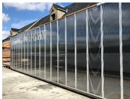
Figure 9: The active façade on the “Living in Light Box”
